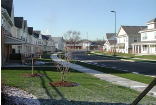
curving street with deflected view
