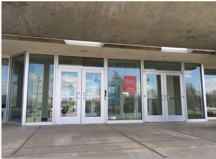
Entrance Door at Wright Hall
