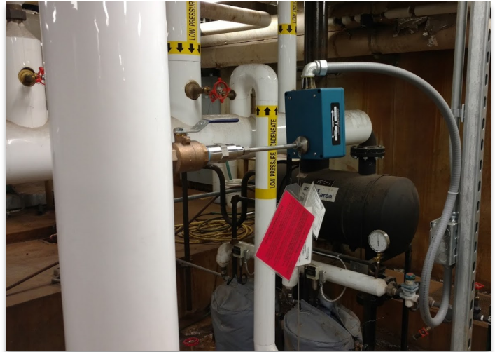
Installation of Condensate Meter at Stevenson Hall
